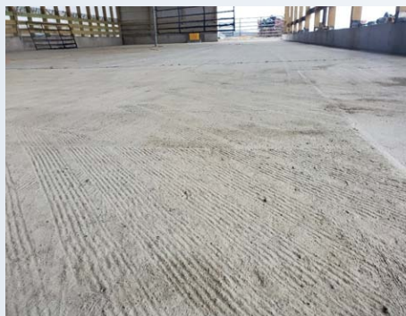
Traction milling technique on the concrete floor.
