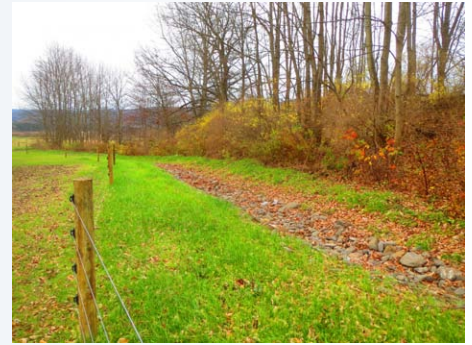
A rock lined waterway with associated livestock exclusion fence installed by Madison County SWCD. This stems soil erosion and improves water quality.
