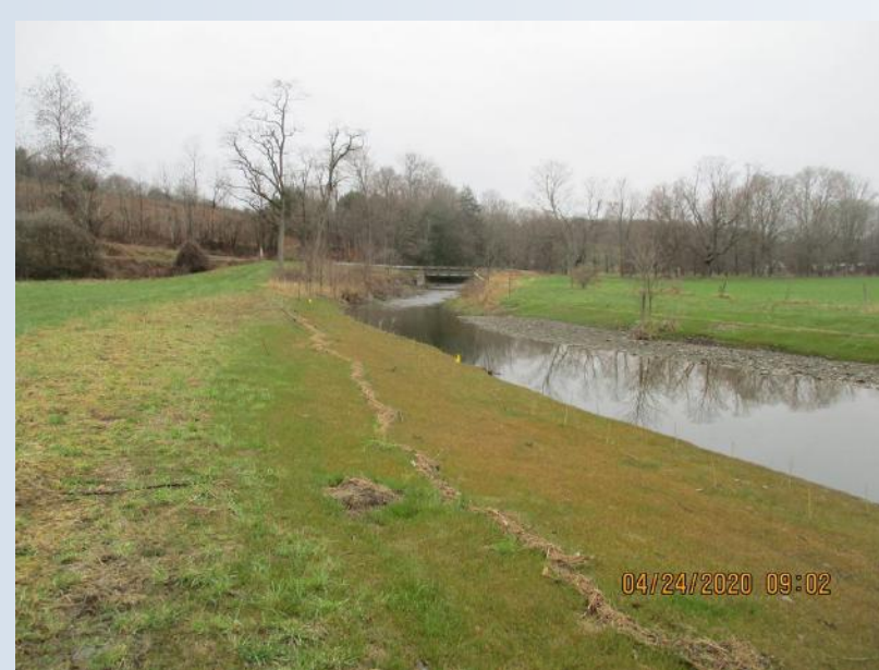
Willow Stakes planted along the Wylie Brook, Photo courtesy Lance Lockwood, Chenango County Soil and Water
