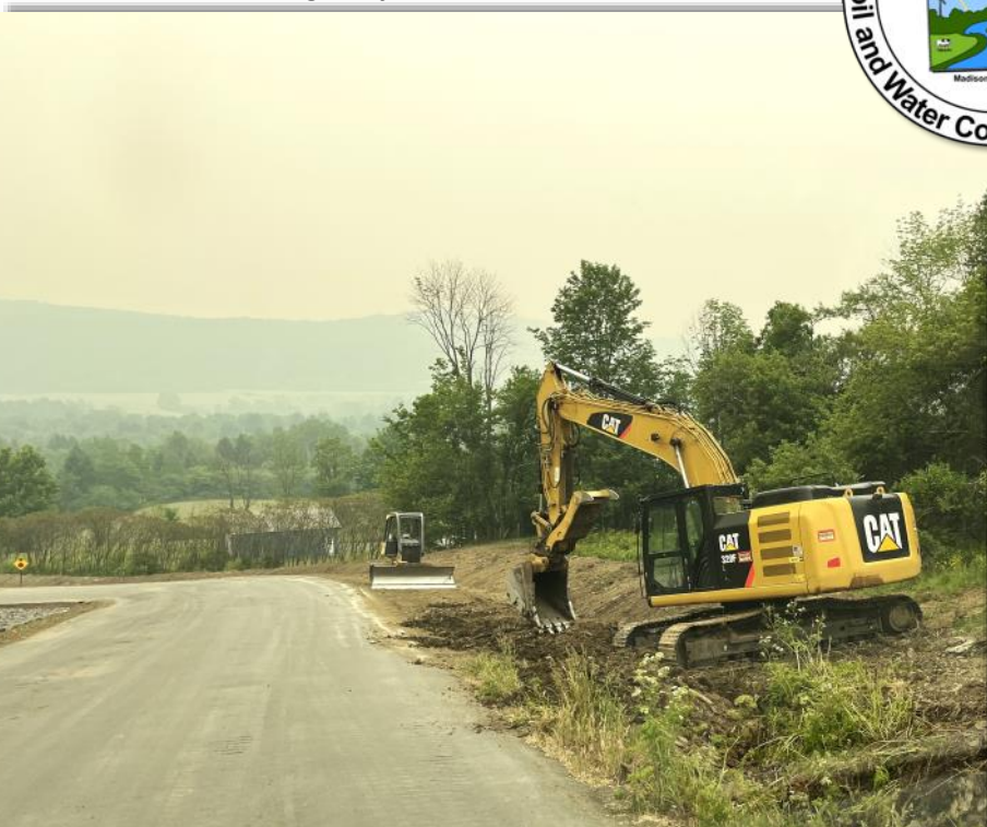
Construction during wildfire smoke
