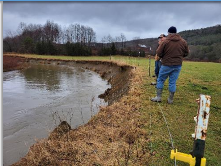
Otego Creek Project 1 streambank erosion before work
