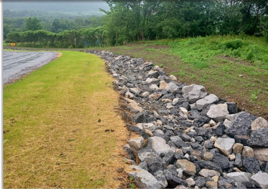
Rock Lined Ditch After Construction
