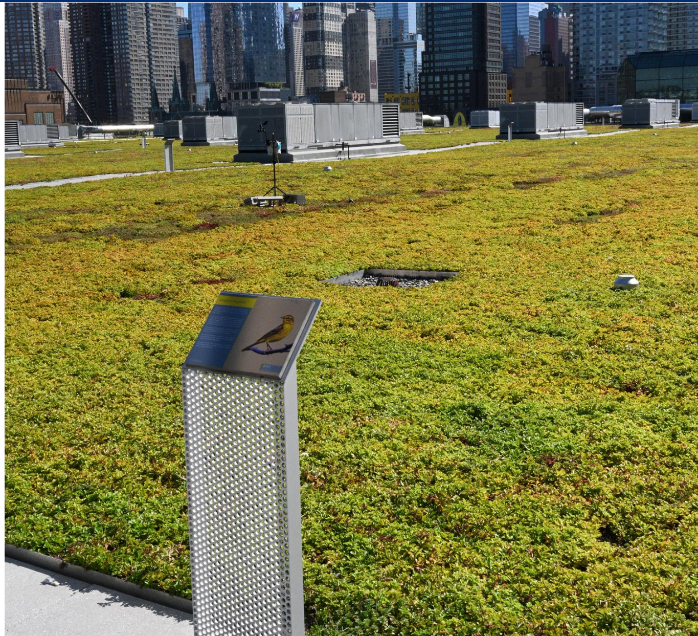
Javits Center Green Roof
