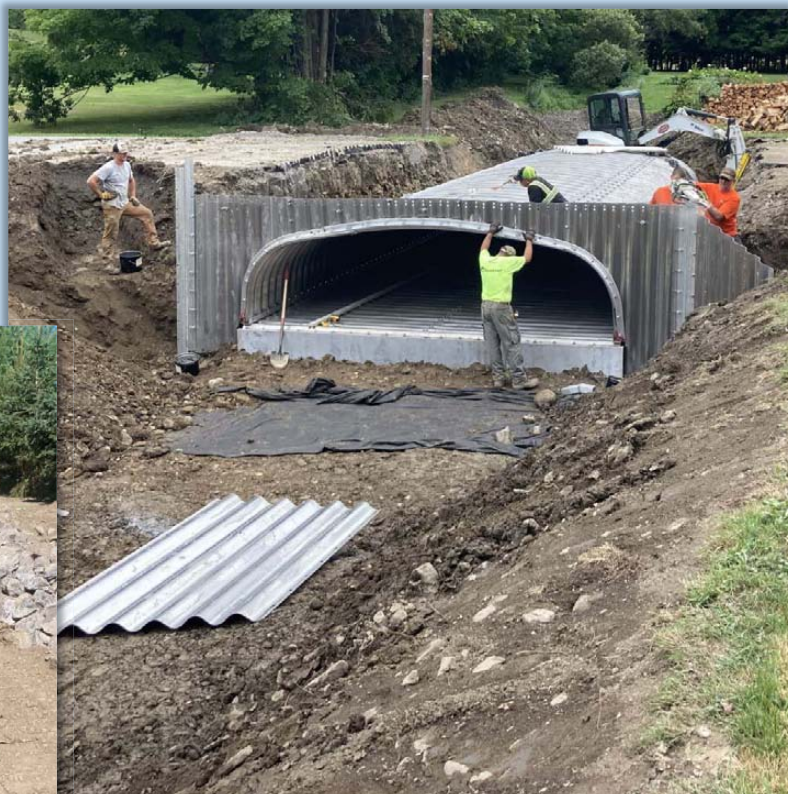
New culvert sized to mitigate road and property flooding issues
