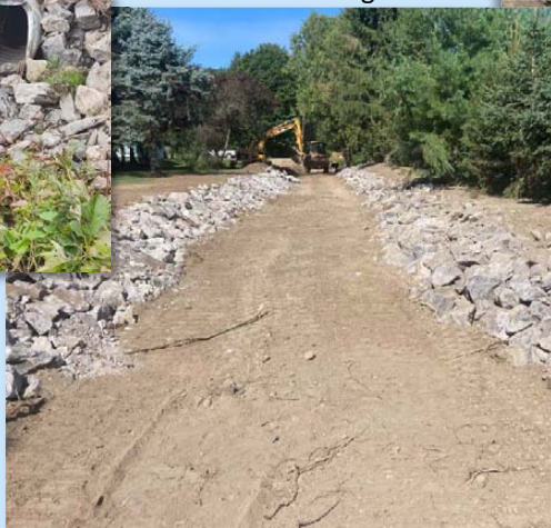
New culvert sized to mitigate road and property flooding issues
