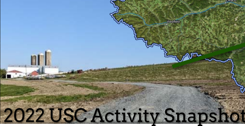
WO Program Project - Tioga County, PA
