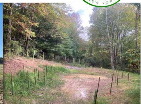
Figure 5: Finished planted stormwater basin at Stoltzfus Farm
