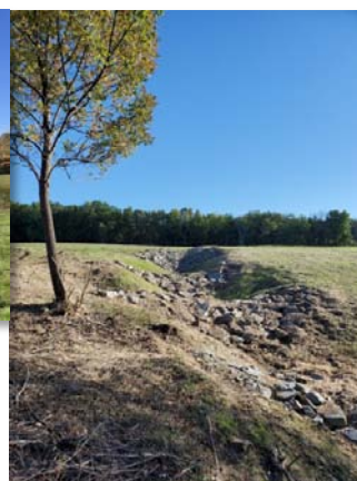
Figure 4: Check dams installed in a tributary that headwaters on the farm
