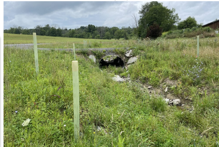
Outlet after stream crossing replacement.
