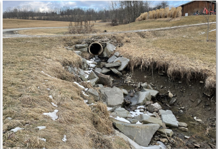
Outlet before stream crossing replacement
