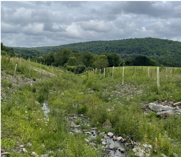
Looking downstream after channel work
