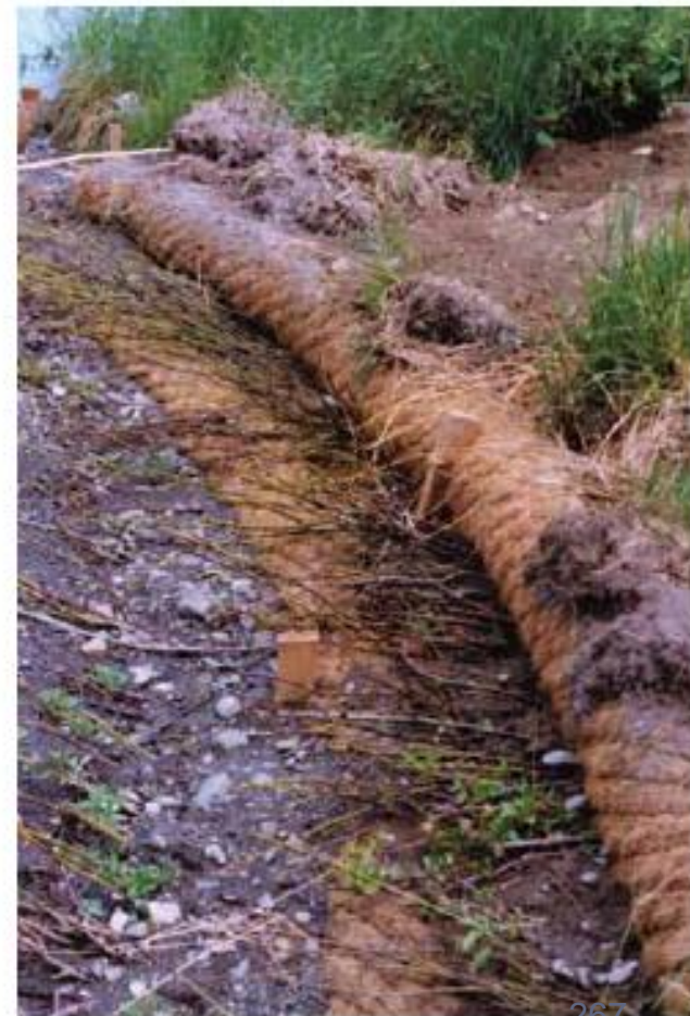
Brush layering with coconut logs.
