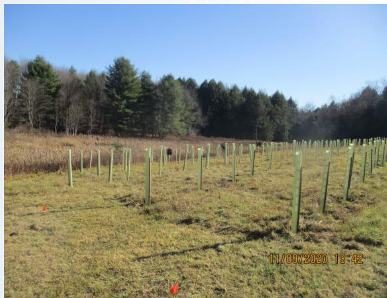
Crew is finishing planting downstream of the pond dike.
