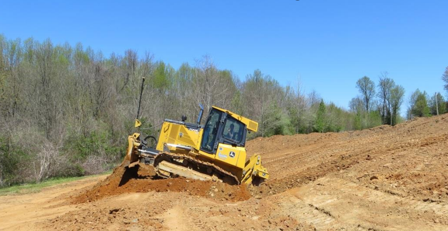
Level-lip spreader during construction
