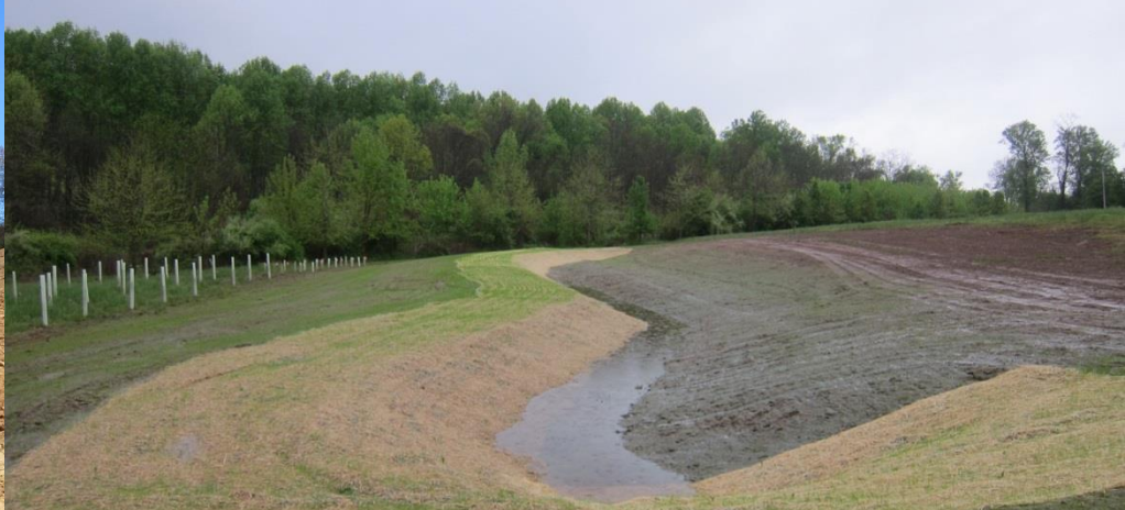
Level lip spreader after construction
