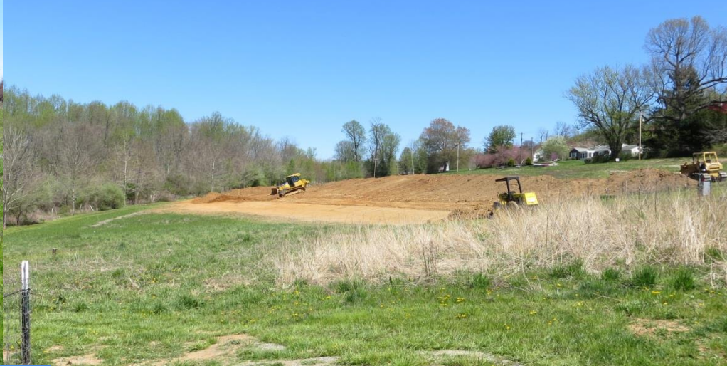
Level-lip spreader during construction
